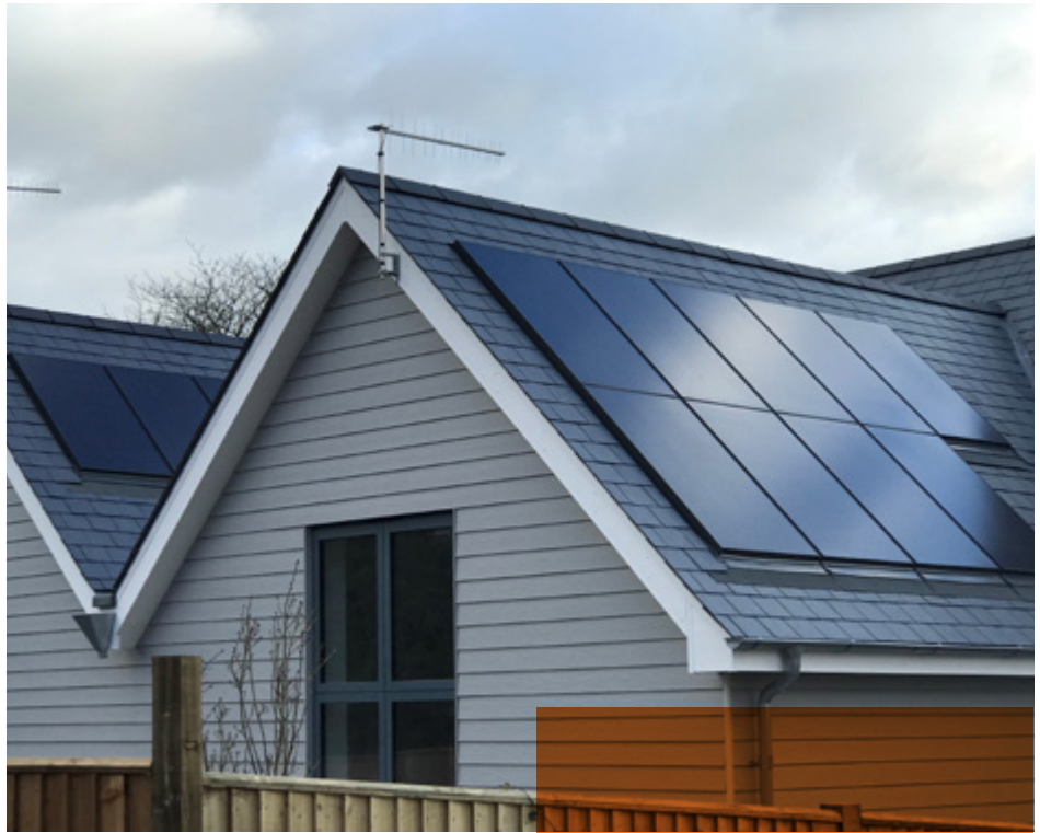
In roof system installed for Millgate Homes
