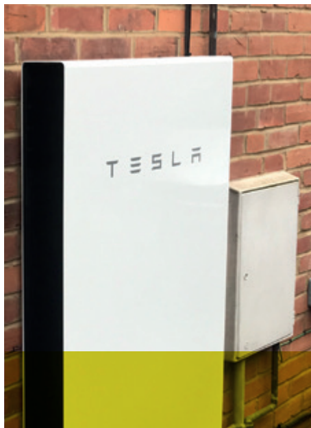
Residential installation of Tesla Powerwall 2
